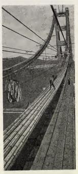
THE ABOVE PHOTOGRAPH SHOWS THE PROCESS USED IN SPINNING THE CABLES ON THE CALIFORNIA BRIDGES, WITH THE CAT-WALK, THE FARTIALLY COMPLETED CABLE, AND THE SPINNING WHEELS—A THREAD—A STRAND—A CABLE.
